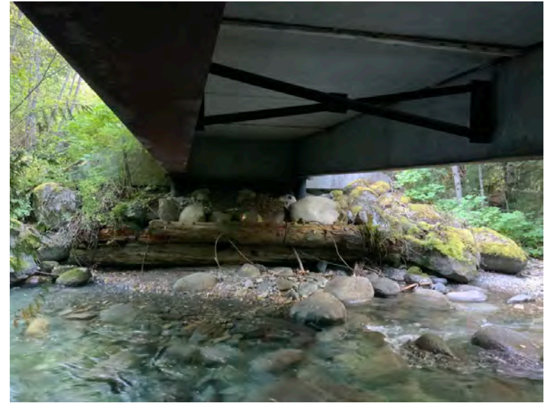
Left Bank Abutment when facing downstream
