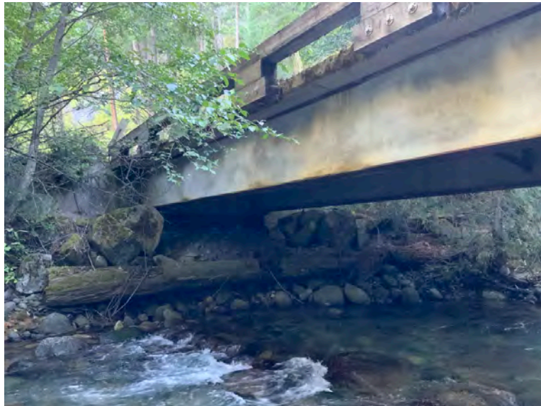
Right Bank Abutment when facing downstream
